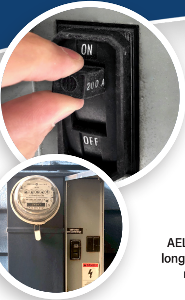
Example of the main shut-off switch at the meter panel.
